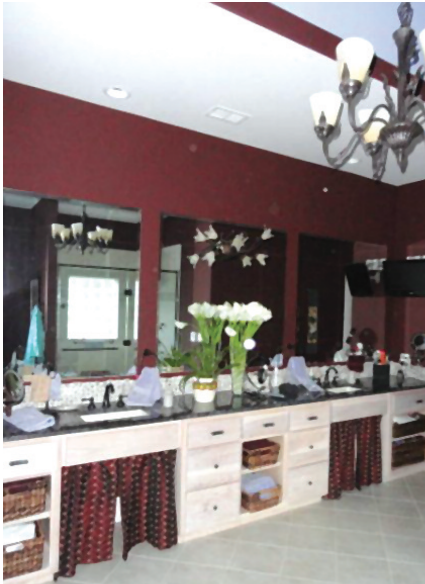
Master bath has knee space under the sinks and a curbless shower (r).
